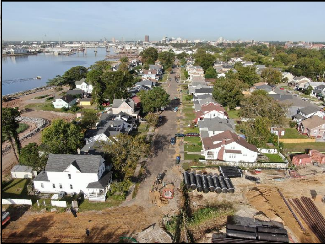
Chesterfield Heights , October, 2020 ~ photo courtesy of MEB General Contractors/ City of Norfolk
